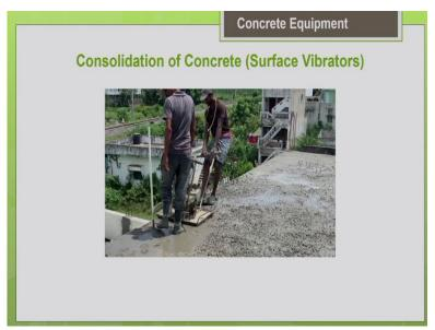
So, this picture also shows how the plate type surface vibrator is used for the slab consolidation.
